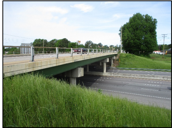
Photo 1 – S-32-273 (Bush River Rd.) Bridge over I-20 in Richland County, SC.
